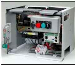
Combination Starter Unit with Circuit Breaker Disconnect
