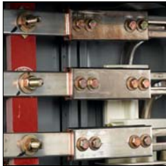
Horizontal Bus Splice
