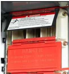
Automatic Vertical Bus Shutter
