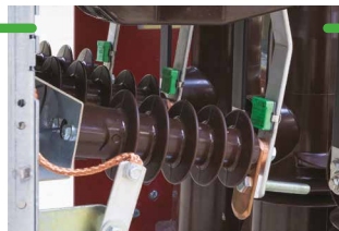
TH110 sensor mounted on cable termination
