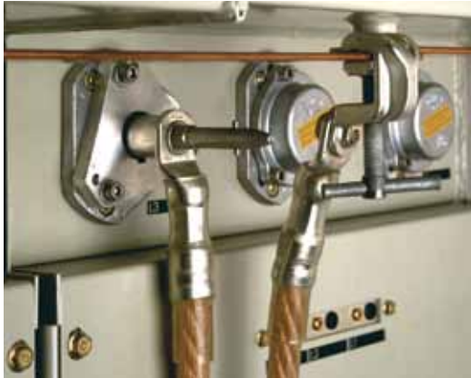
System earthing and earthing for work purposes
