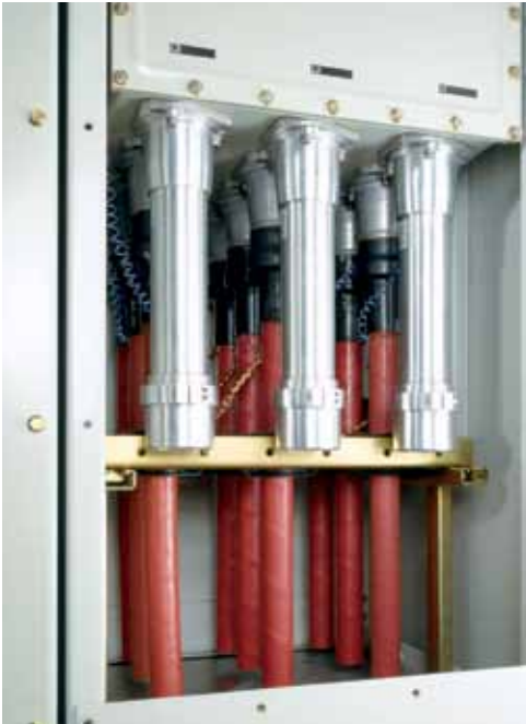
Cable connection compartment with surge arresters and multiple cable connection
