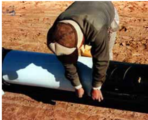
Insulrap 50 being installed insulation
