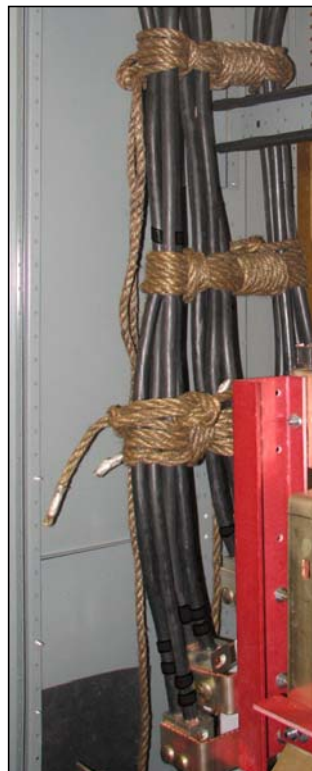
Figure 25 – Cable Restraint Example
